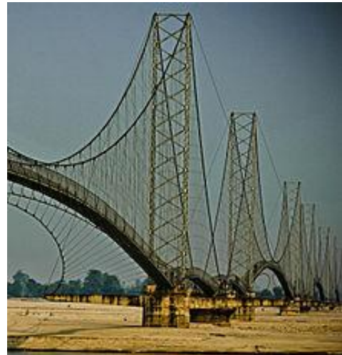
Dodhara Chandni Bridge over Mahakali river
