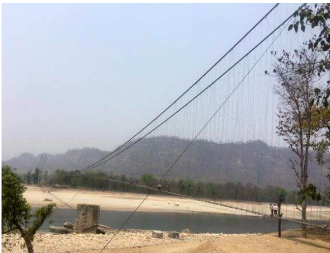
Ghatghaon Bridge in Surkhet
