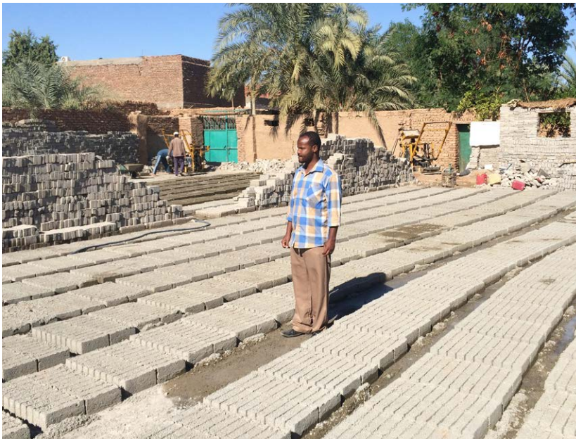
A villager helps make bricks to repair irrigation canals. © SDC
