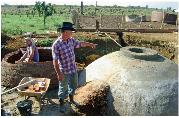
Cuban smallholder farmers take advantage of biogas plants to dispose of their pig slurry and generate gas for their own use
