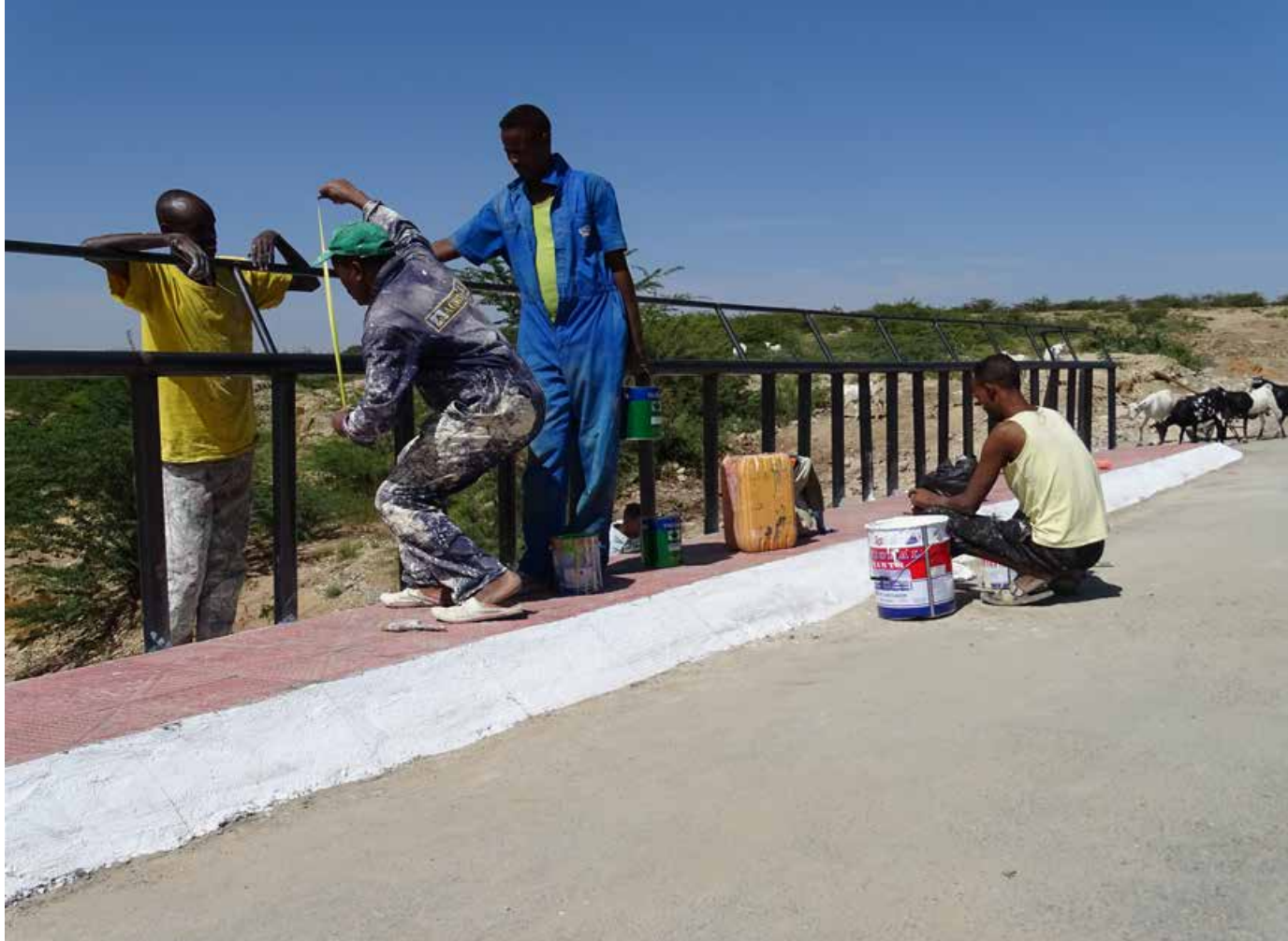
Road work with support from the Local Development Fund
