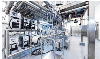
Givaudan and Bühler jointly run the Apac Protein Innovation Centre, a 400-square-metre facility at Givaudan's Woodlands site. PHOTO: GIVAUDAN SINGAPORE
