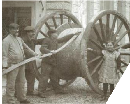
Foundation of FATZER AG
