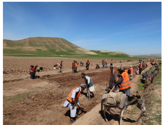
Ongoing construction works, Rustaq, Takhar Province, 2017, © SDC.
